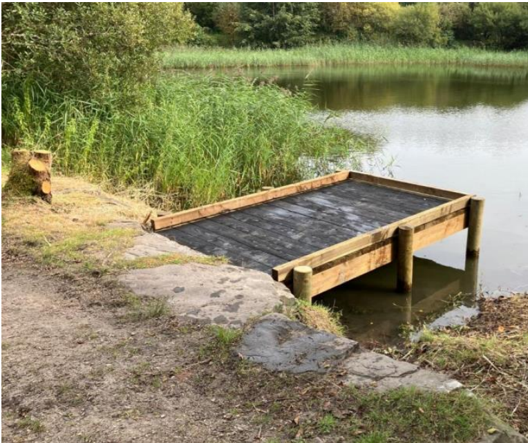
Angling platform constructed at Morolwg Pond, Carmarthenshire
